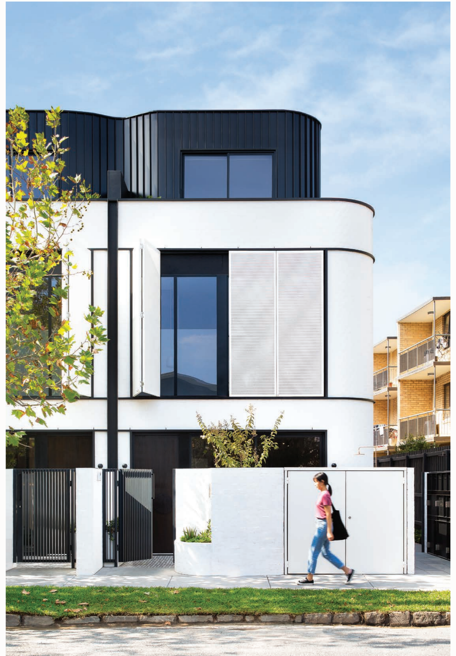
PAST PROJECT - PINE AVE, ELWOOD
